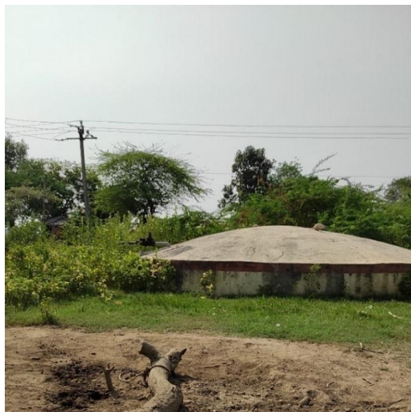
(F-4.4B-RO water plant)
