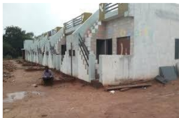
(F-12.6.J-kolavada in house condition)
