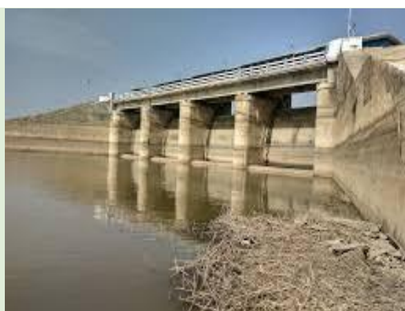
(F-12.6.P-budhel in dam)
